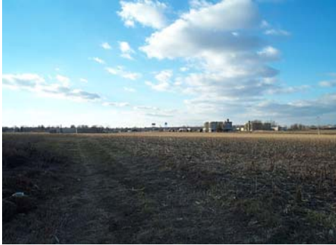
Water Treatment Facilities on East Approach
